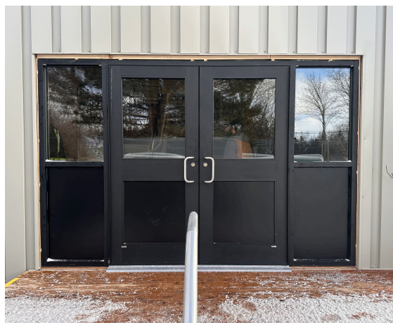
Just installed and ready for final trim!
